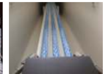
Whisper quiet linear winches use composite rope which is quieter and stronger than steel cable
